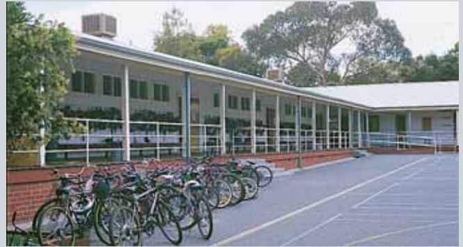
6 units installed at Coolbinia Primary School, Perth Western Australia.
